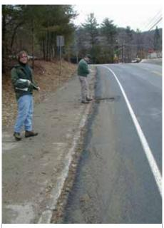
Photo 13: Beach Road showing sand buildup from winter sanding operations
