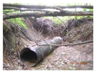
Photo 12: Erosion at the Exit 21 tributary (looking upstream)
