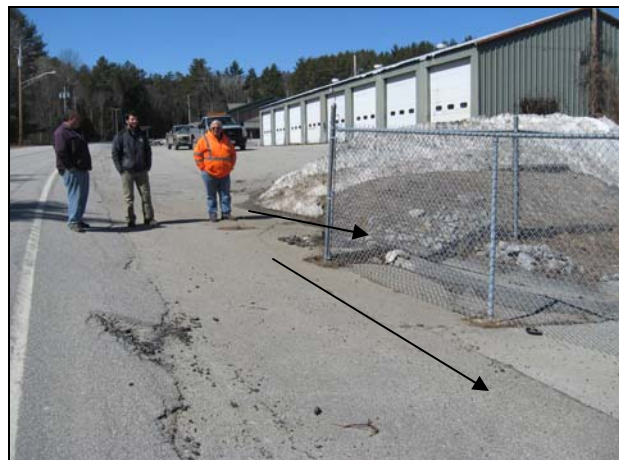
Stormwater Drainage from Lake Shore Drive to the Old Highway Garage
