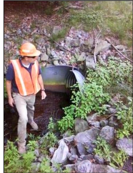
Paved Ditch to Finkle Brook On Valley Woods Road
