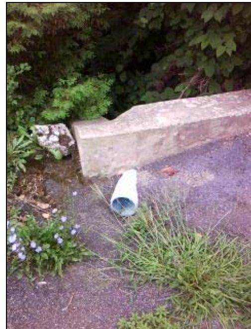
The North Side of Goodman Avenue Draining to Stewart Brook
