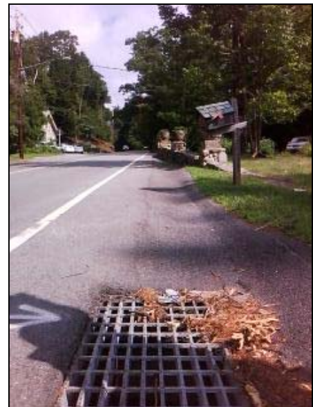
Paved Ditch to Drop Inlet on Lake Shore Drive
