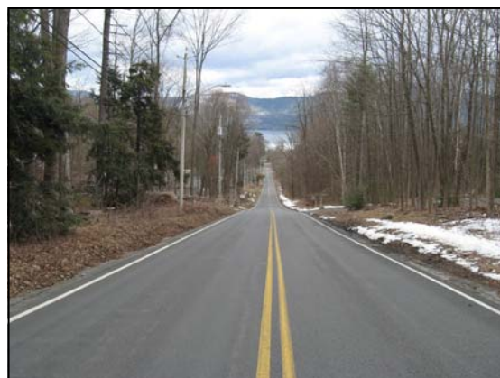
Mohican Road Drainage
