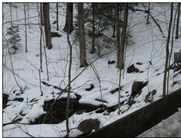
Frank Cameron Road Culverts
