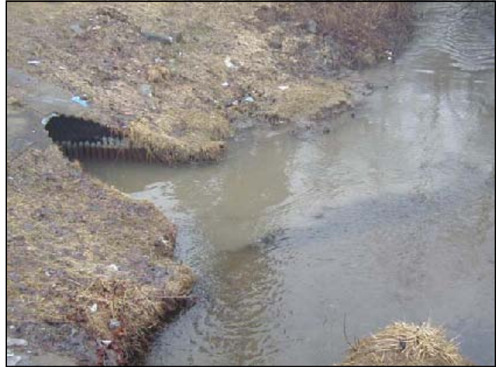
Stormwater outfall entering trout stream during a rainfall event
