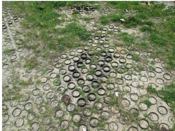
Figure 3.9.2. A Level 3 investigation is warranted if more than 25% of the permeable pavement surface appears to be clogged, or joints are filled in, or, as shown in the photo, vegetation is growing.
