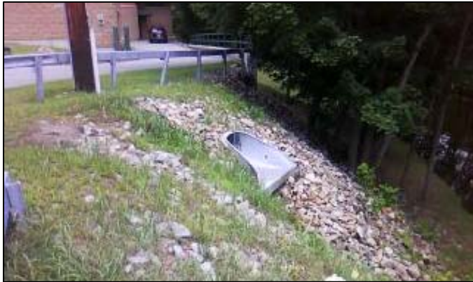
Outfall from Main Street to North Creek
