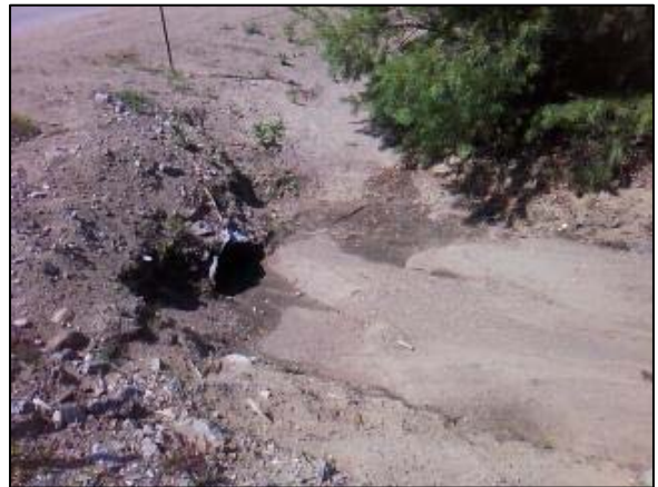
Route 28: Eroding roadside ditches
