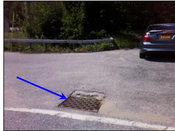
Intersection of Ski Bowl Rd & Main St: Drop inlet conveys directly to tributary
