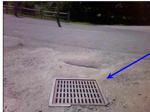
Intersection of Main St & Railroad Place: Drop inlet that outfalls to tributary
