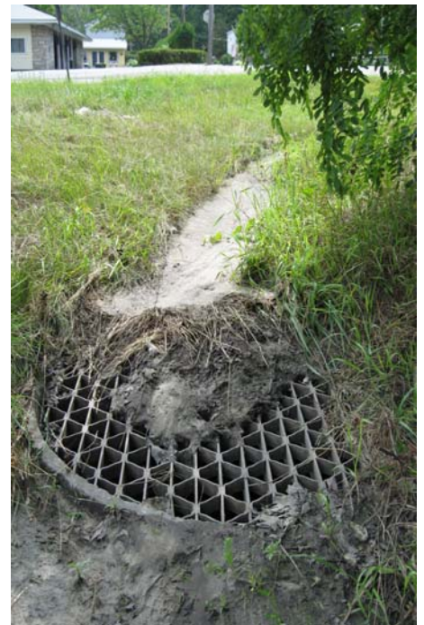
Drop Inlet at Exit 22 & Rt 9
