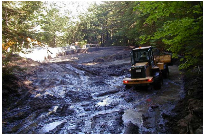
Cleaning out Hubble Reservoir in 1999
