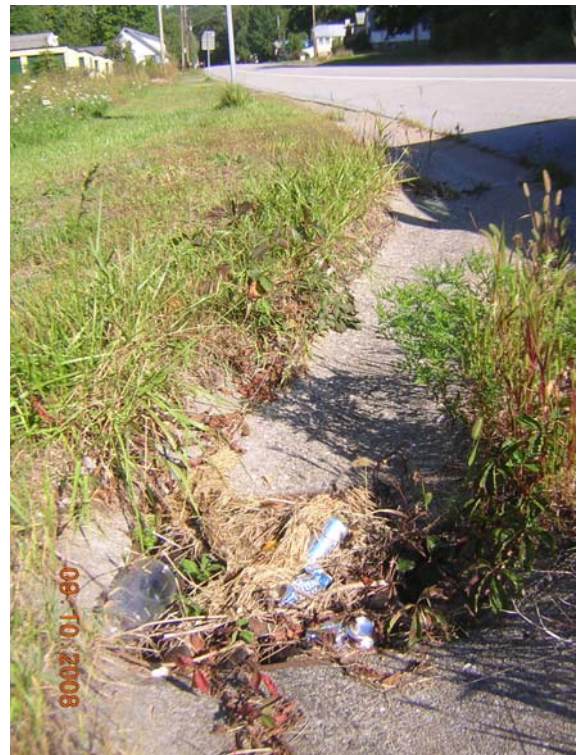
Drop inlet along NYS Route 9 which is plugged with garbage and debris. These locations are excellent candidates for stormwater retrofits
