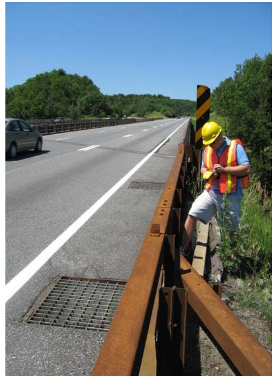
Drop inlets on I87 which drain directly down to NYS Route 9 and then into English Brook
