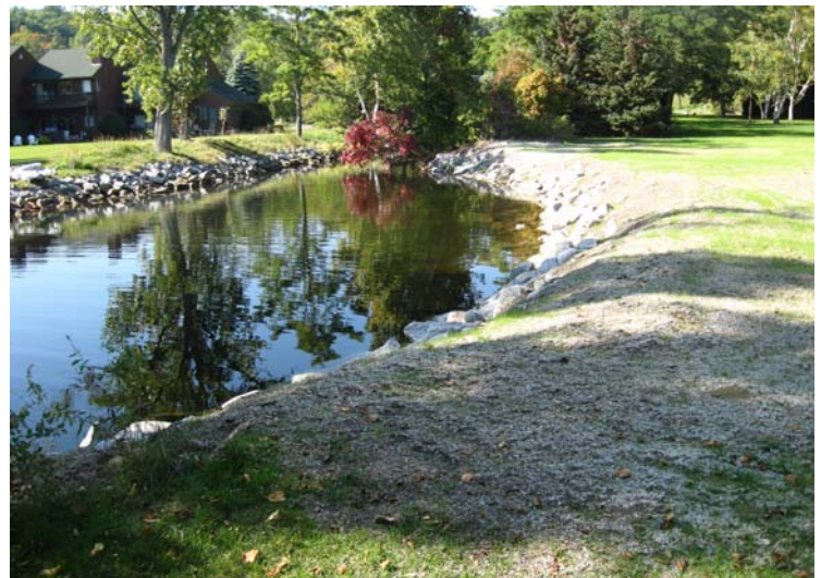
Hague Brook in-stream sediment pond on Lake George Land Conservancy property, created in 2007. This picture is taken one week following seeding. This basin collected more than 250 tons of sediment and debris in one year.
