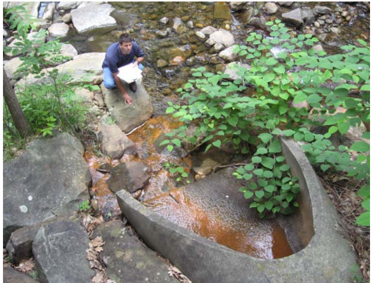
Large stormwater outfall from Exit 22
