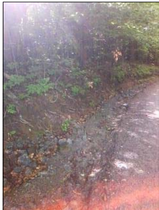
Location 2: Burnt Hill Road ditch before intersection with Hayesburg Road
