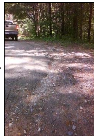
Crystal Lake Road erosion
