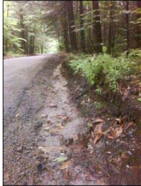
Location 1: Burnt Hill Road ditch erosion
