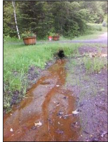
Burnt Hill Road intersection: ditch to stream & lake
