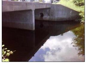
Route 9 Outlet: Stormwater conveyance to Chester Creek
