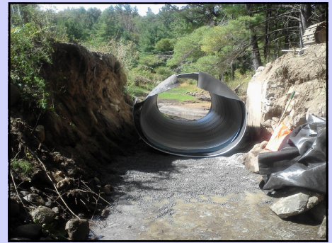
Battle Hill Road crossing during construction
