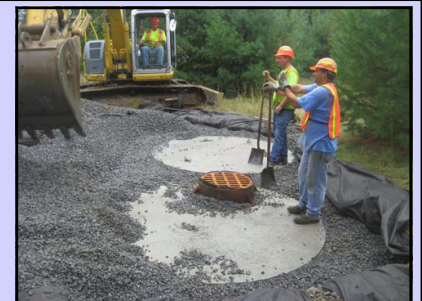
Project during construction
