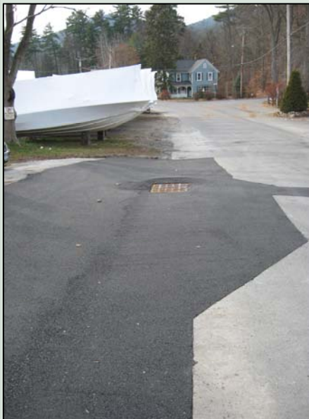
Paved swale to convey stormwater
