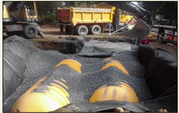
Infiltration chamber installation
