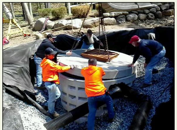
Drywell installation
