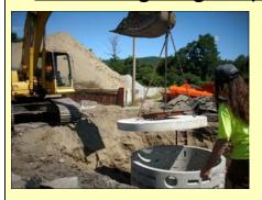
In the summer of 2010, the Warren County SWCD and Town of Lake George Highway Department completed a significant stormwater infiltration project at the town's highway facility. This system was designed by the District and treats all stormwater runoff from the totally impervious 2+ acre town highway property, eliminating a huge source of sediment and pollutants flowing into the adjacent waterbody, West Brook.
