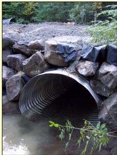
pipes aren't cheap (\$100+ per foot just for the pipe), so the town highway departments were thrilled to get all materials paid for through the grant. All culverts replaced were structurally failing, and the towns would have had to pay for these replacements themselves in a few years anyway. So, not only did this project work out for improved fish habitat,
