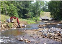
With such limited funding, the District rented an excavator and bulldozer and conducted all of the construction efforts with its staff. Over the period of 3-4 weeks, all work was completed for this restoration project, including new fish habitat improvement structures in the brook. The Districts hope that this 500 foot section will be used as a demonstration area for future restoration efforts on this stream.
