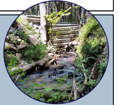
Buckbee Road pre construction
