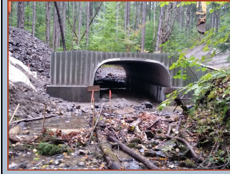
....the new properly sized structure
