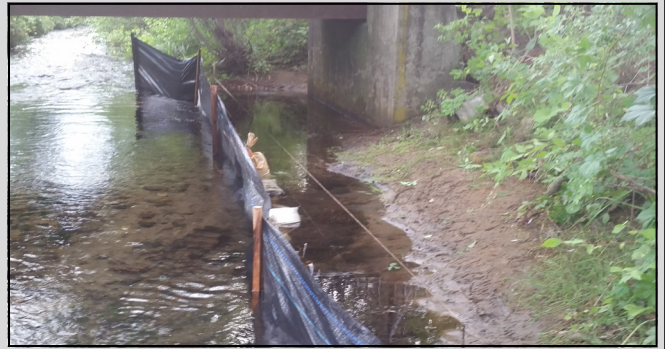
Pre-construction on the West Brook
