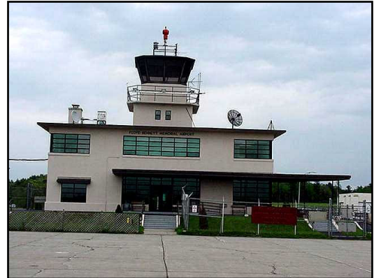
Photo – 5 Terminal Building
