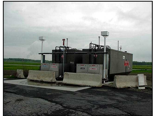
Photo 4 – Fuel Storage Facilities
