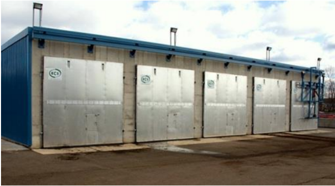
Figure 3-10 Example Containerized In-Vessel Aerated Static Pile
