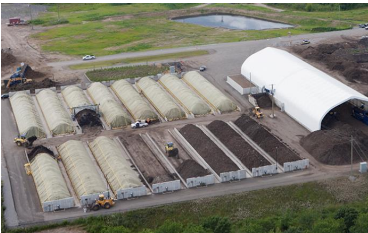
Figure 3-11 Example Covered Aerated Static Pile (C-ASP) Facility
