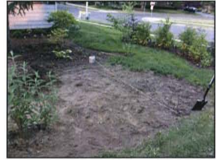
Area measured to get sense of natural slope and needed height of berm.
