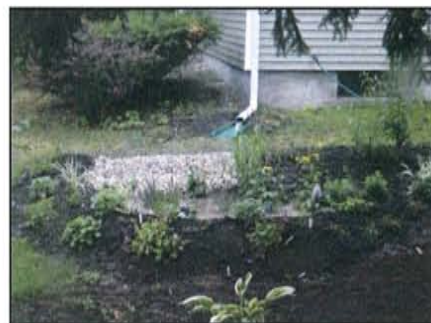
Neighbor (grey house) installs new gutter, downspout, and splash block. First rain.
