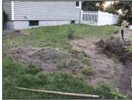
Owner of white house builds rain garden. First, garden area is scraped of grass and weeds.
