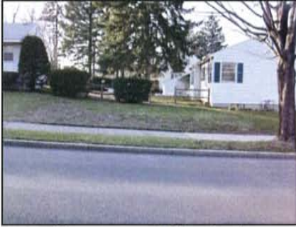
Runoff from property on left (grey house) creates large puddle in backyard of white house (right). Rain garden site is between the two houses, on the slope.
