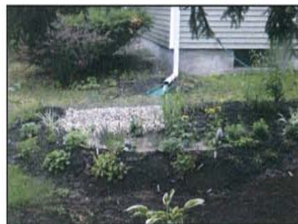
Neighbor (grey house) installs new gutter, downspout, and splash block. First rain.
