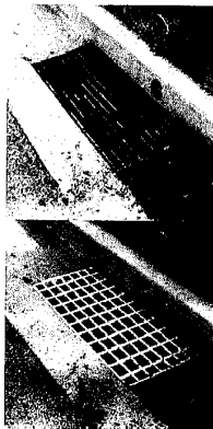
Figure 10 - Above, poor drainage grate choice; Below, bicycle-friendly grate (photos courtesy of Syrcast)
