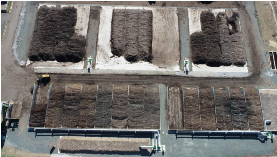
Figure 3-7 Example of Reversing Extended ASP Primary and Walled Secondary (80,000 tons per year capacity)
